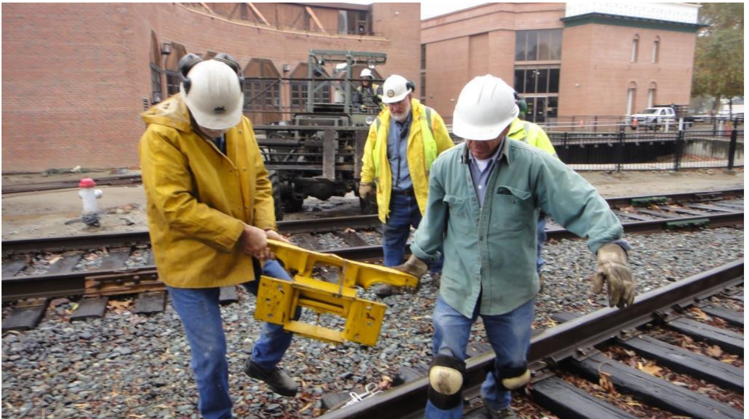
Alan and Mike T. bring the new derail into place
