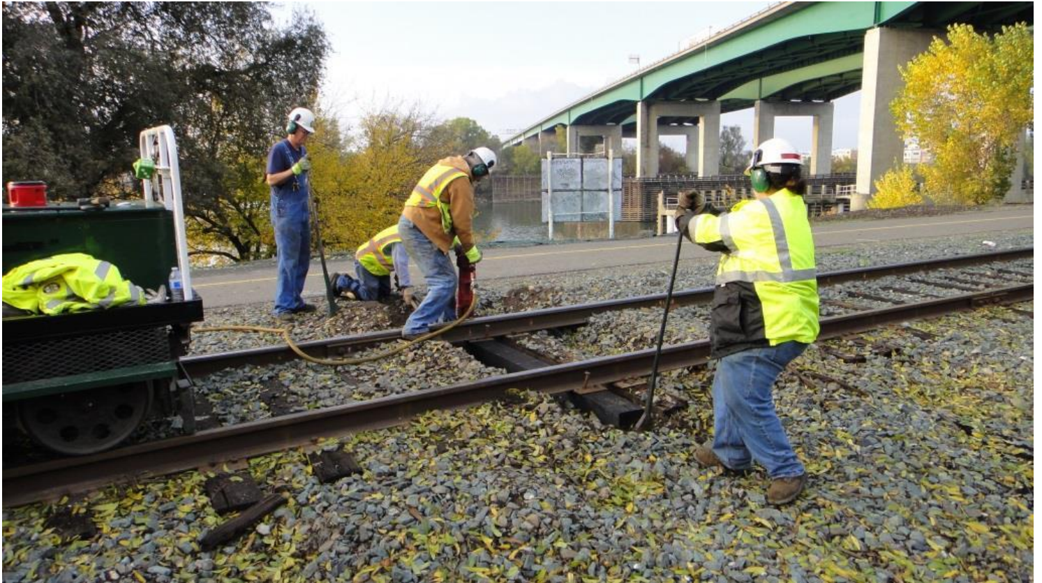
Steve uses the pneumatic spiker while Heather nips the tie
