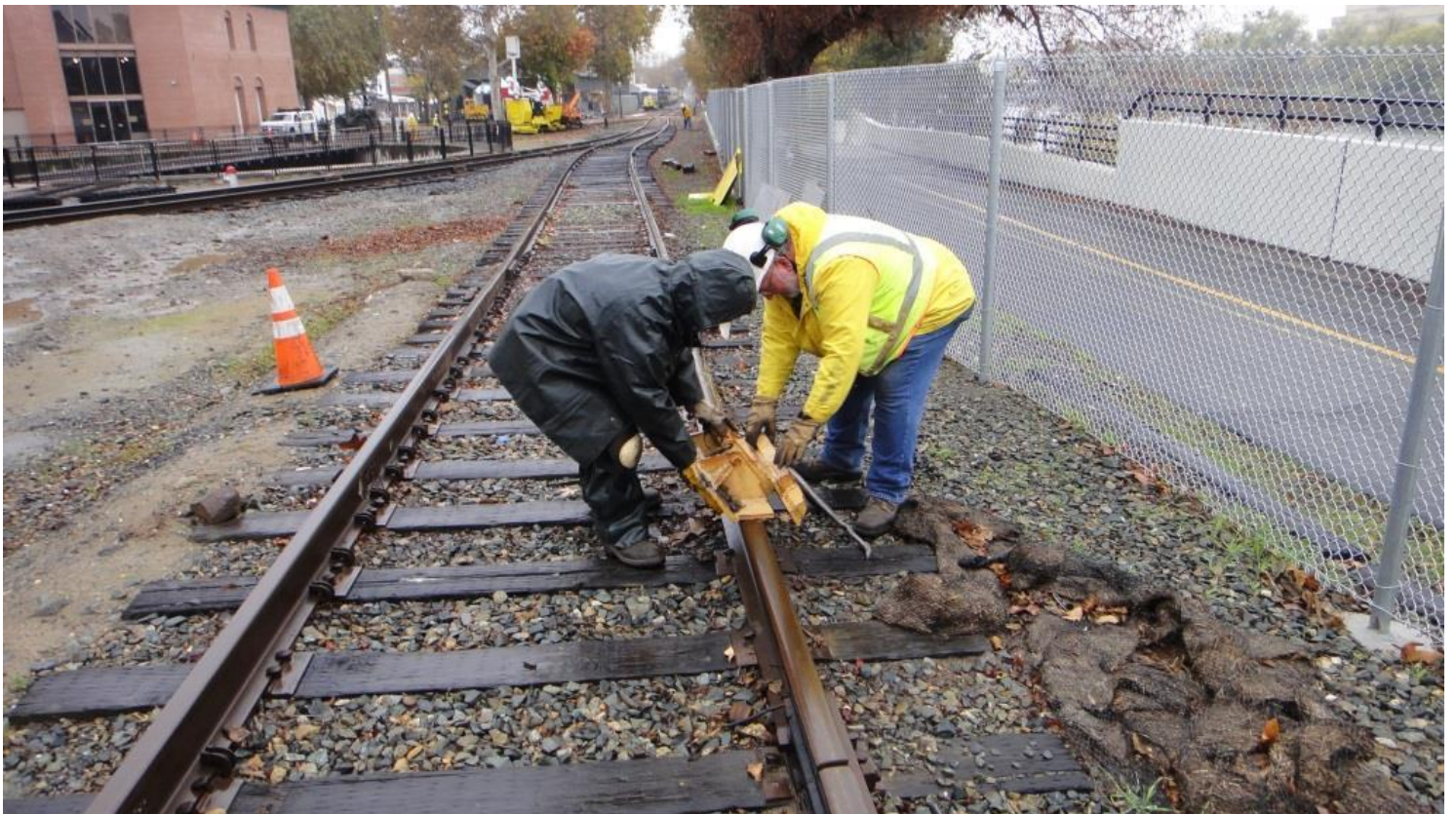
Mike T. and Frank slide the old derailed into a new position
