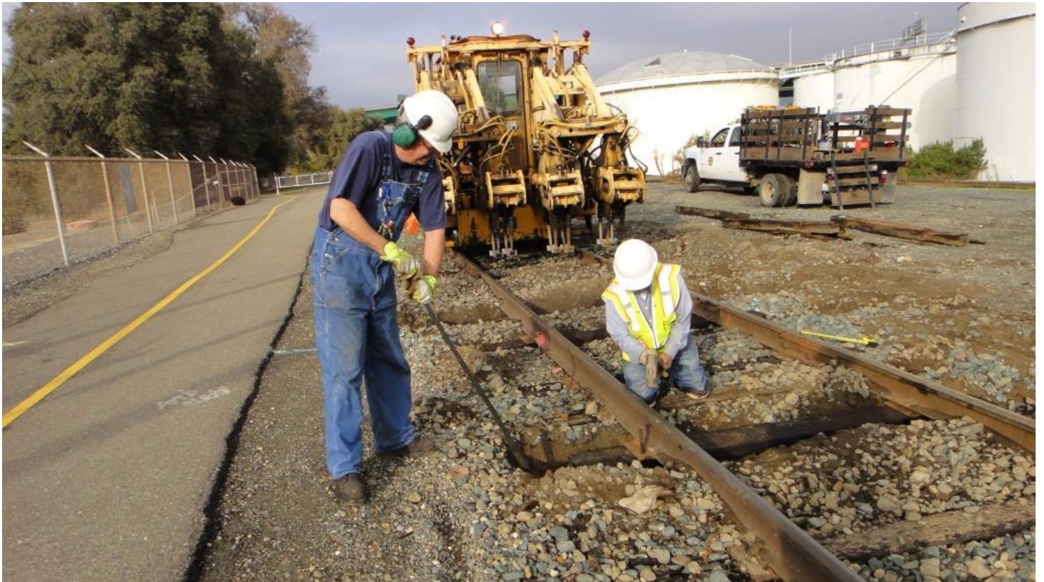
The serious work at hand, Dave nips the tie while Mike T. sets spikes
