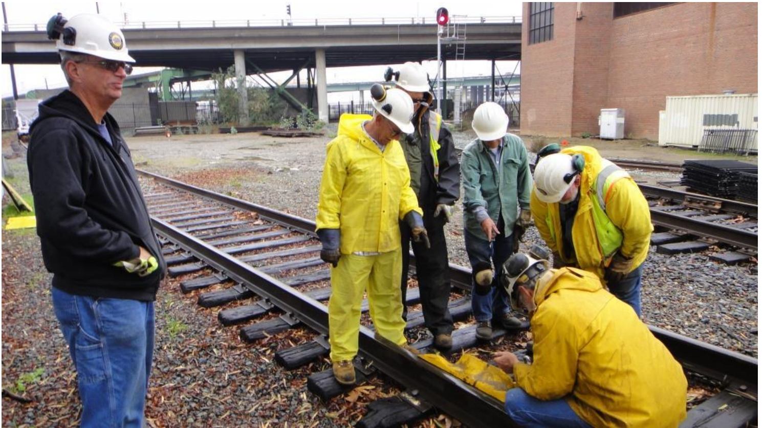
How many Maintenance of Way volunteers does it take to install a derail?
