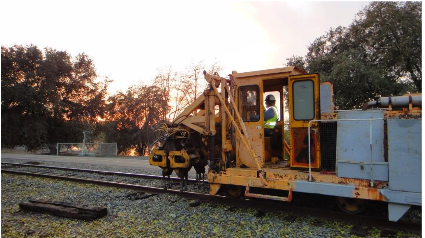
Tamping the track at sunset...
