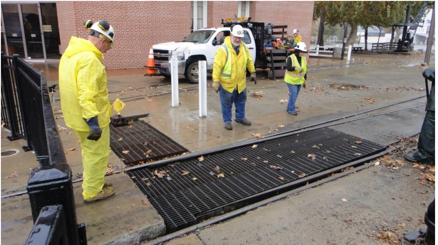
Clem, Frank, and Pam admire the new grating in place
