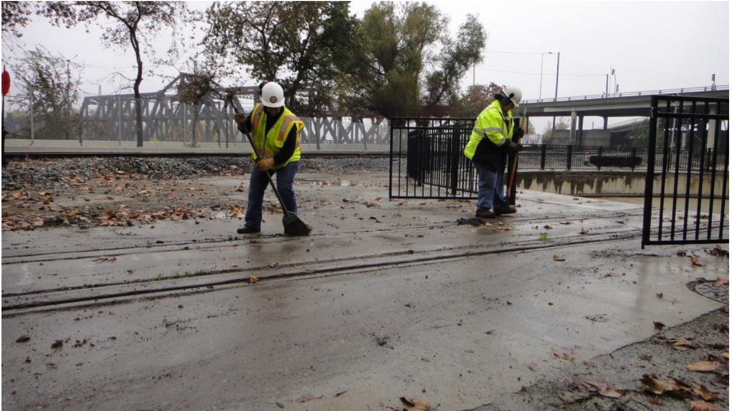
Pam and Heather clear out the flange-ways on the North Turntable Lead
